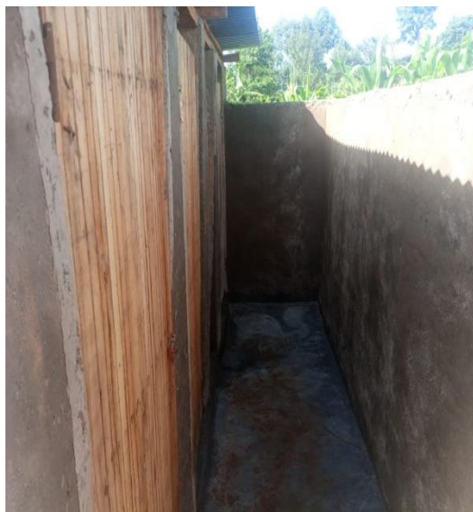
New Latrine with brick walls and stucco overlay
