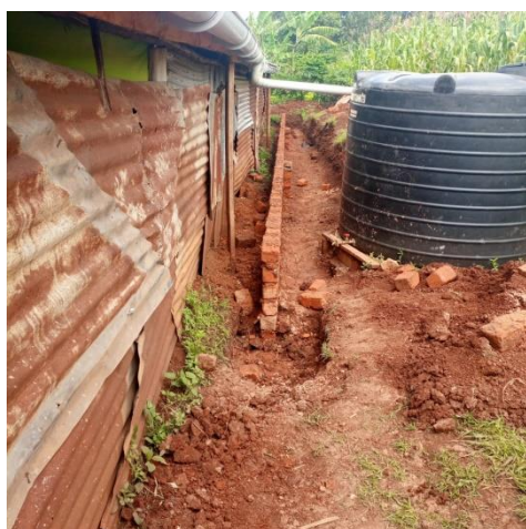
New Wall along the Church with Water Tank
