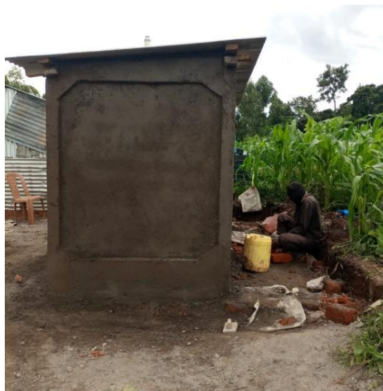
New Latrine with brick walls and stucco overlay
